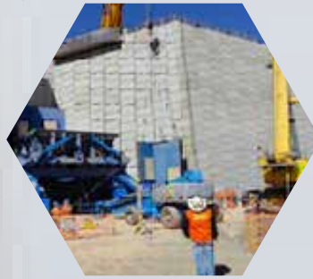
Inspection of Contruction Reinforced Earth Wall
